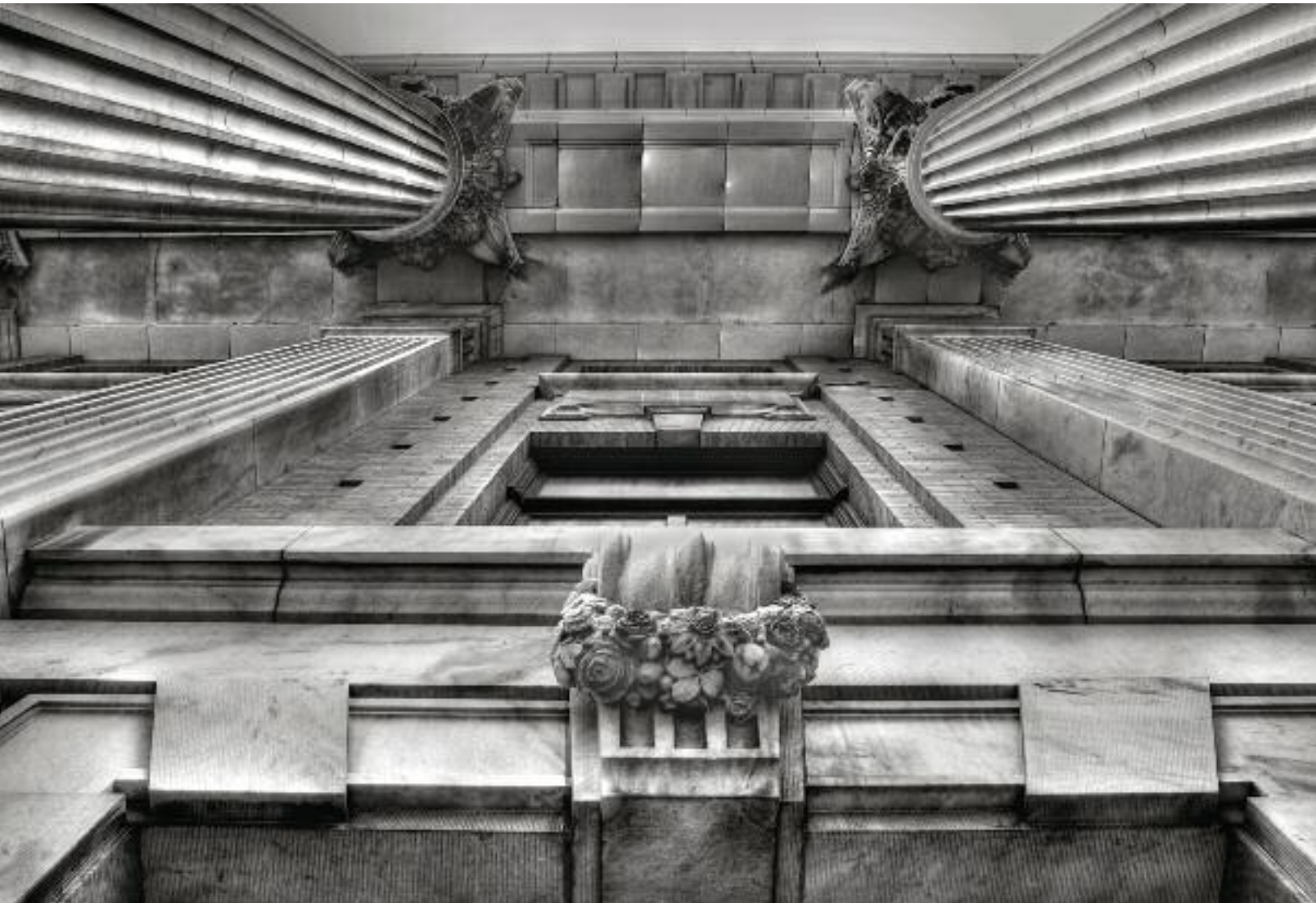
This is the old Federal Court House in Tampa.
