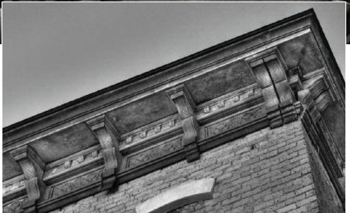
The Fitzgerald Building is the oldest surviving business structure in the Port of Tampa.
